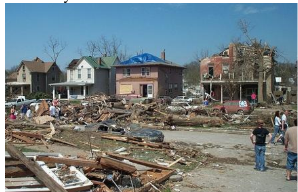
Figure 1. Iowa City, 14 April 2006. A high-end F2 tornado ravaged part of the downtown with numerous roofs tore off, overturned cars, and scattered debris. Photographer: unknown.
