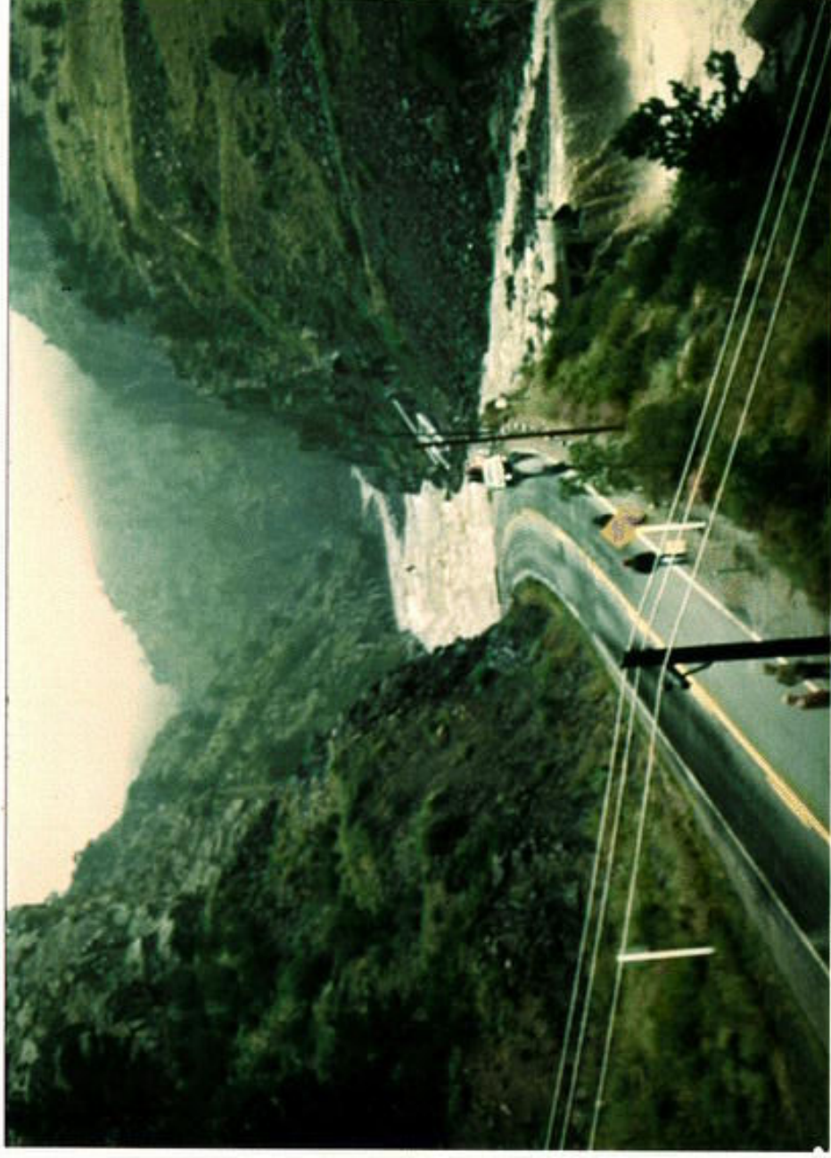
ID. BIG THOMPSON CANYON FLOOD no. 34ct! Mouth of Big Thompson Canyon looking upstream into Narrows. Highway 34 at left, truncated by river. Preliminary calculated peak discharge at this point was 31,200 cubic feet per second. Larimer County, Colorado. August 1, 1976.
