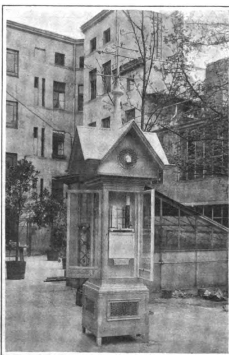
Fig. 3.—A well-constructed German kiosk.
