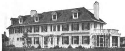
All walls coated with Trus-Con Stone-Tex
